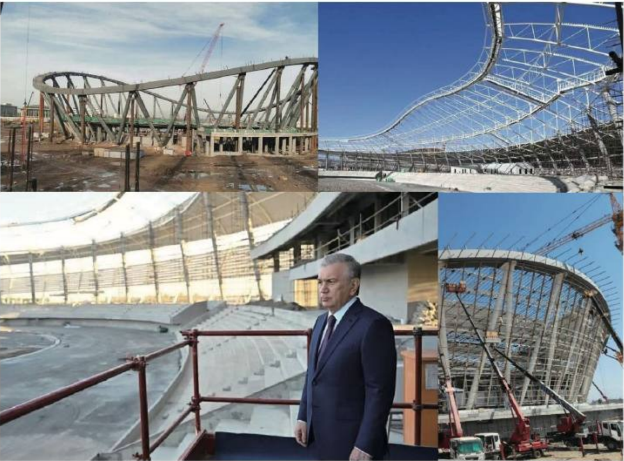
The President of Uzbekistan visiting the construction site.
